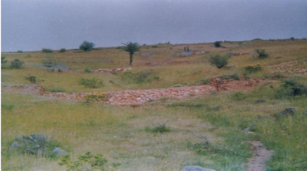
Fig. 34.5 Loose boulder check dam for gully erosion control
