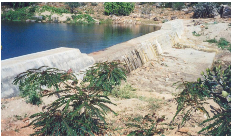
Fig. 34.4. Concrete check dam for gully control
